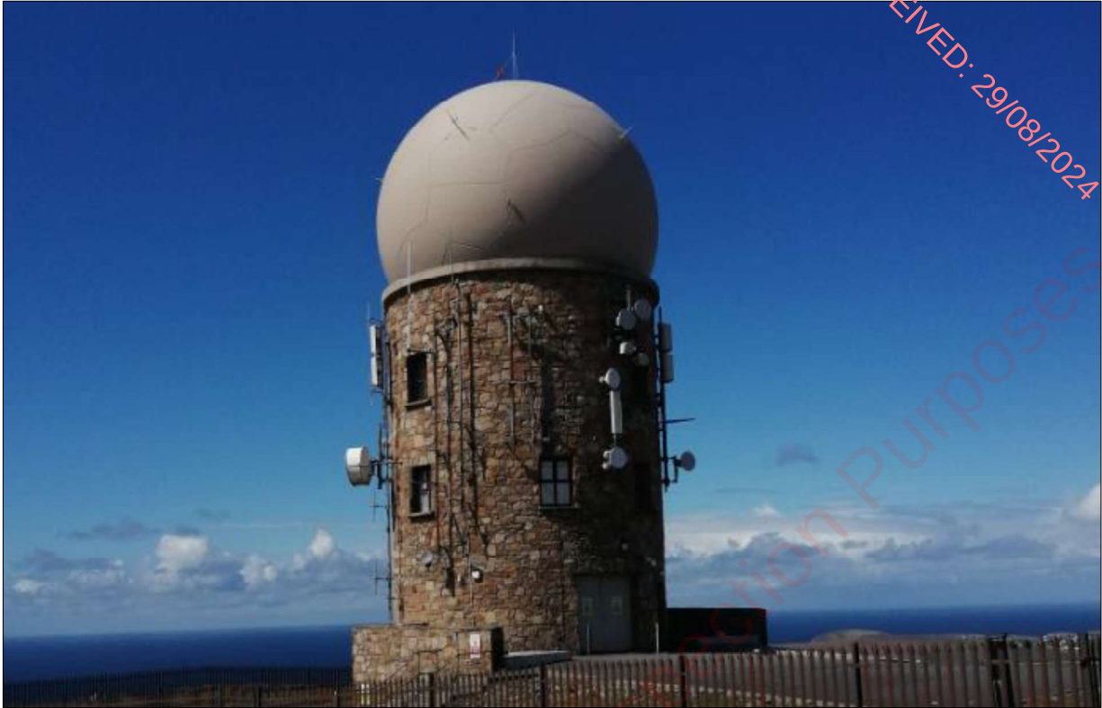
Figure 9.1. IAA Radar Surveillance Site – Dooncarton
